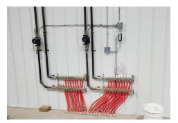
DGH completed design for hydronic in-floor heating to provide more comfortable heating during Manitoban winters
